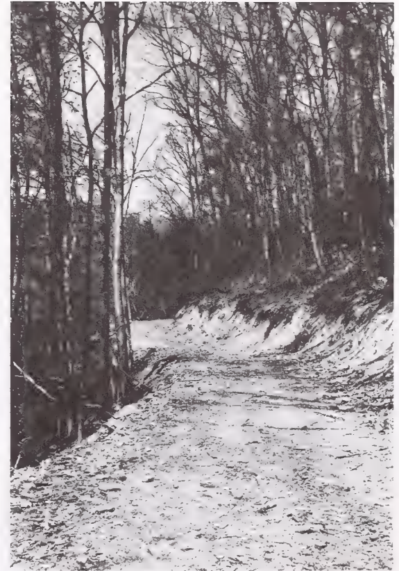
Low-cost, low-maintenance forest roads can be designed and built with features that protect water resources from unnecessary siltation.
